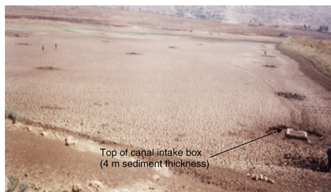
Fig. 2. Adikenafiz reservoir. The top of the inlet canal is clogged due to excessive sediment deposition and is shown cleared from sediment.
